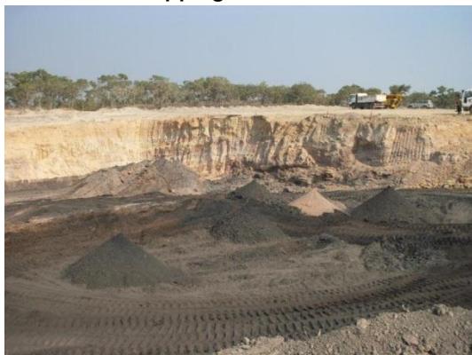
Pre-Stripping at Mbalawala
